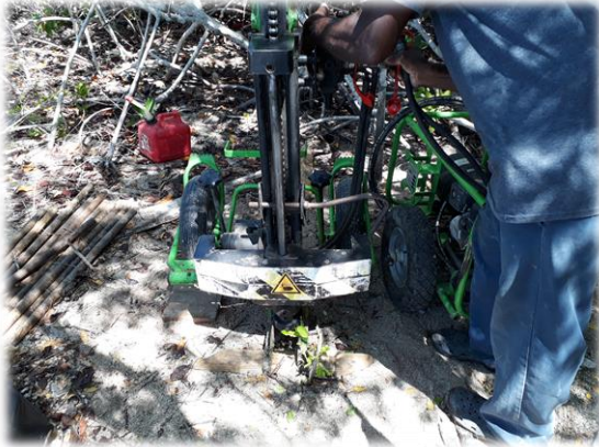
Attaching pipes to being driven @ BH1
