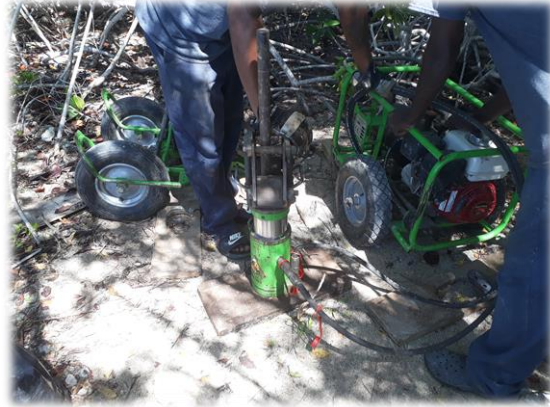
Extracting pipes after test @ BH1
