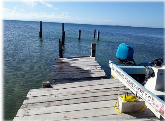
Small pier at Twin Caye
