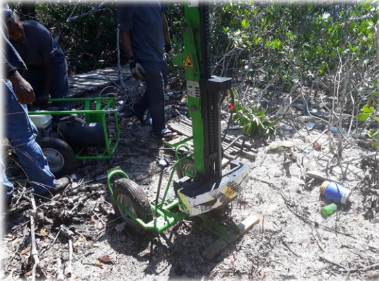
Attaching pipes to being driven @ BH2
